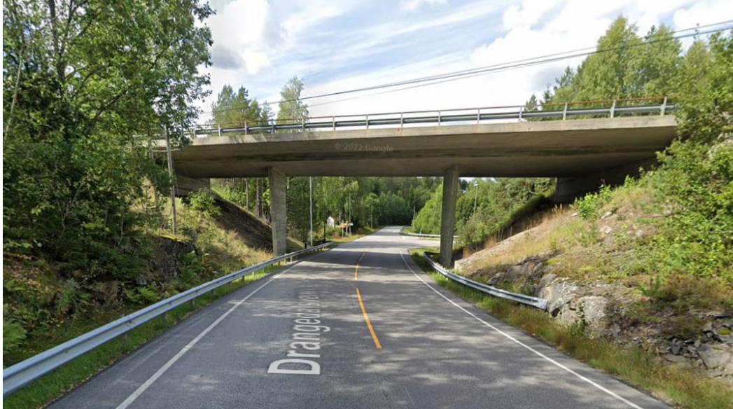
Figur 3-14: 08-0919 Gjerdemyra bru. (Foto: Google Street view).
