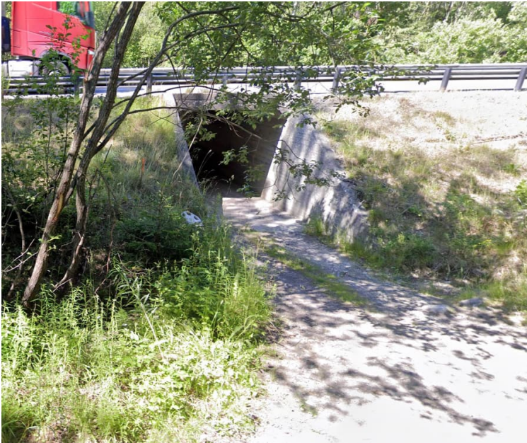
Figur 3-8: Eks kulvert. (Foto: Google street view).
