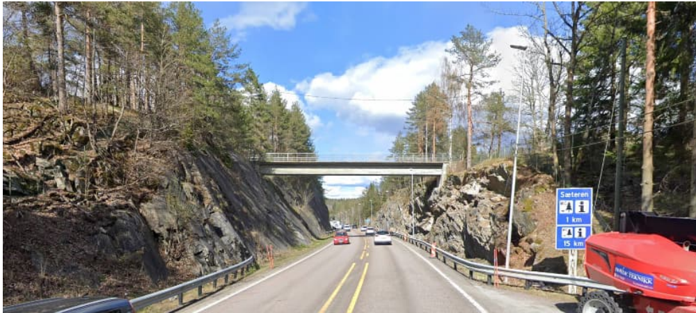
Figur 3-33: 08-0784 Skauen bru. (Foto: Google Street view).
