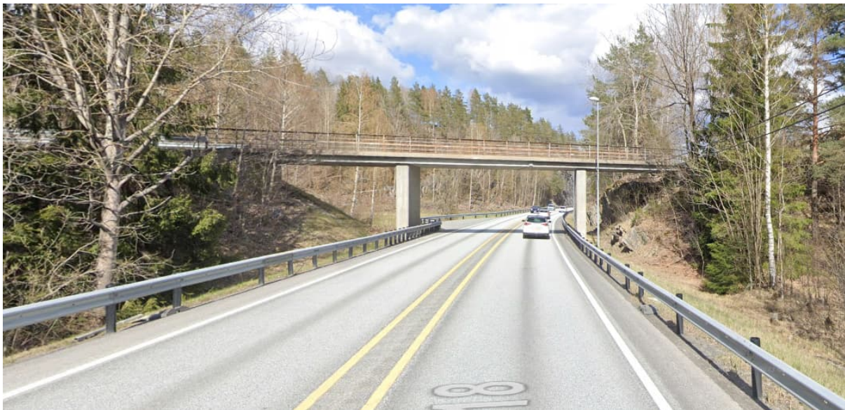
Figur 3-34: 08-0763 Setern bru. (Foto: Google Street view).
